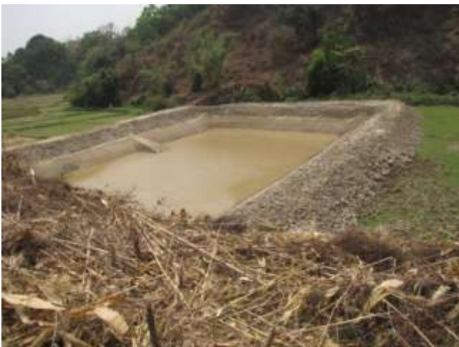
Water harvesting structure with fish at NAIP site
